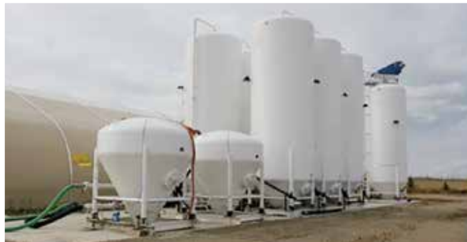
2014 Wilco Bulk Cement Plant | Williston, ND, USA (May)
