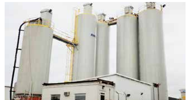
2 – BMH Systems Concrete Batch Plants Closes: 5/15 Contact: Harris Houston +1.770.304.3355
