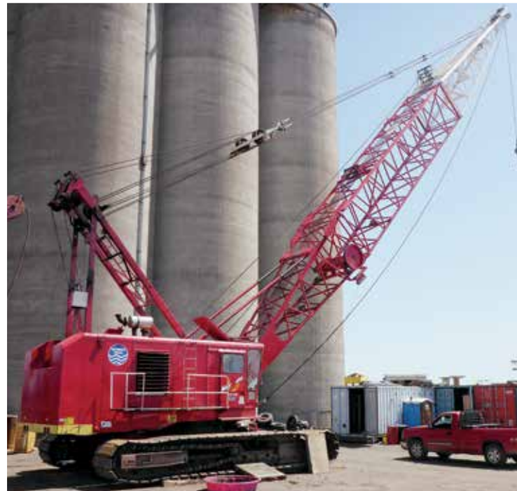
Manitowoc 4100W | Chicago, IL, USA
