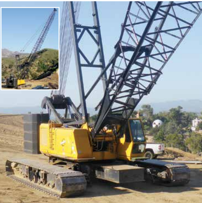
Manitowoc 888 Series 1 & 2 230 Ton Self Erecting | Los Angeles, CA, USA
