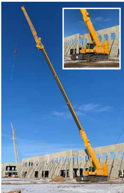
Liebherr LTR1100 110 Ton Rocky Mountain Regional Event
