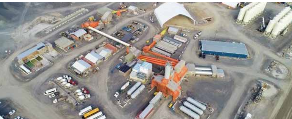
Erie Twin Drum Concrete Plant | Gillam, MB, CAN
