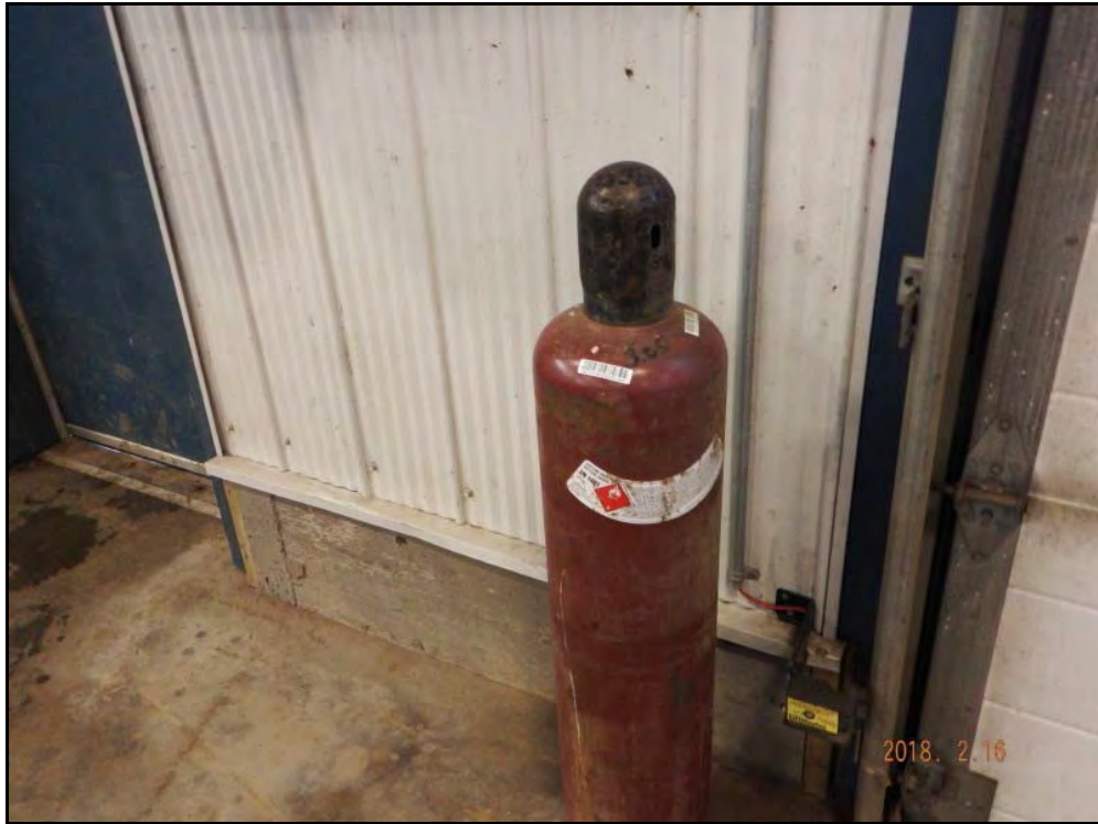
Photograph 33: Compressed air cylinder stored within the shop.
