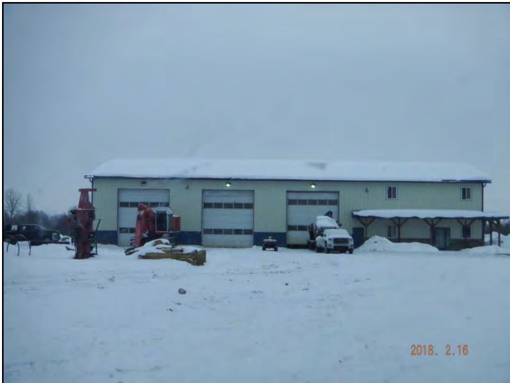
Photograph 5: North-facing view of the building.
