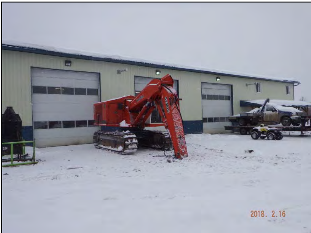
Photograph 8: Northeast-facing view of the south side of the building.
