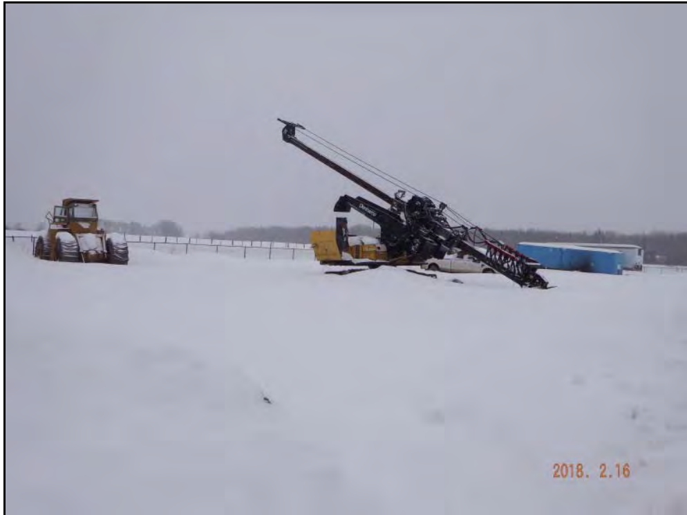
Photograph 21: Southeast-facing view of the eastern side of the yard.
