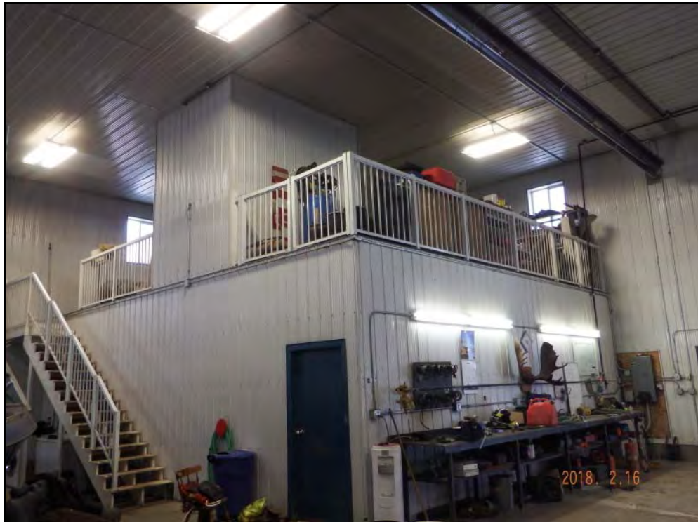
Photograph 28: View of the loft observed within the shop.
