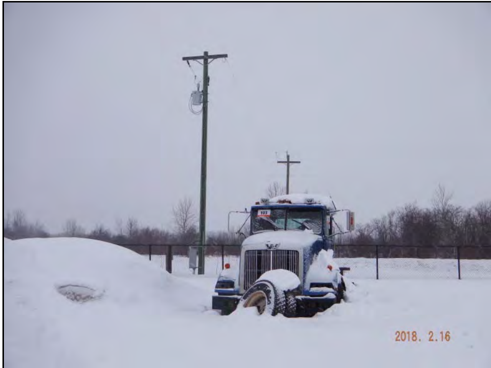
Photograph 11: Transformer observed north of the Property.
