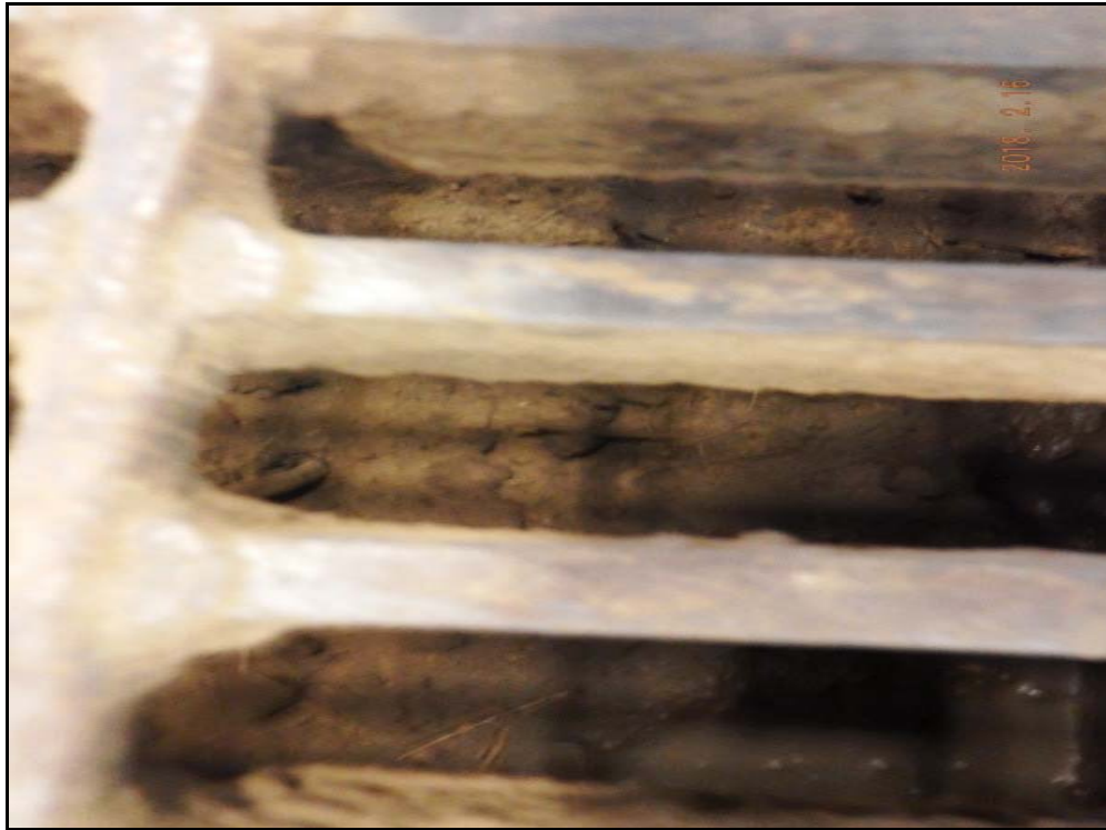
Photograph 37: View of dry drain system observed within the shop.
